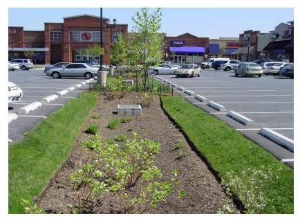
Figure 13: Bioretention BMP
